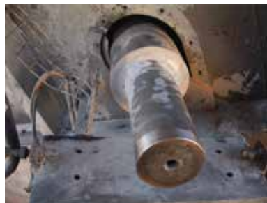
A Perfect Finish! And ready for work again by the end of the shutdown!
