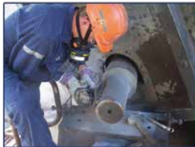
After building up the shaft with Belzona 1111, the former is removed, and the excess Belzona ground off
