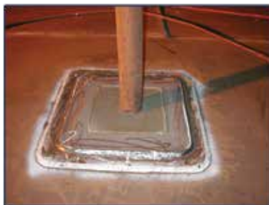
Pad in Position
