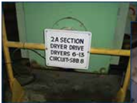
Location of Shaft to be Repaired
