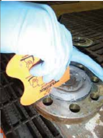
Belzona® 1111 Supermetal being applied
