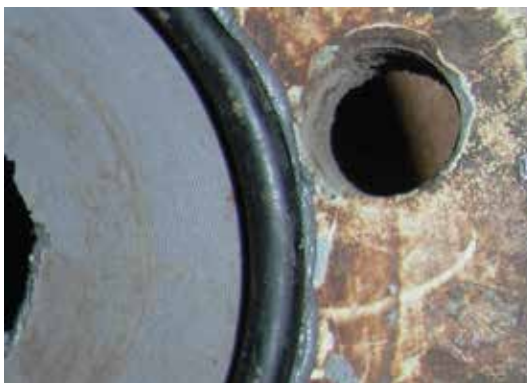
Completed application (before O ring removed) and edge cleaned up
