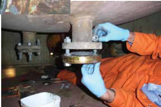
Completed application (before O ring removed) and edge cleaned up
