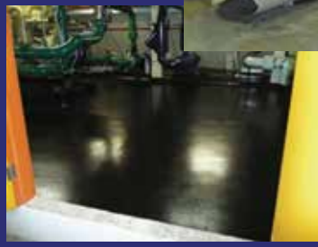
Old vinyl flooring in the plant room.
