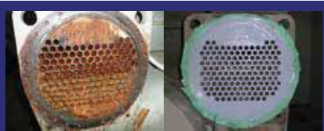
Air conditioning chiller before & after... What a transformation!
