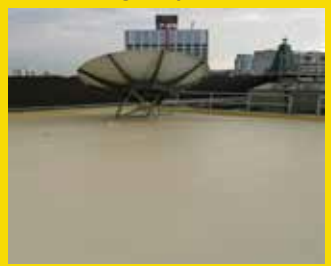
Fully refurbished roof... better than new!
