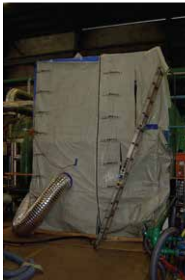
Containment for Sponge-Jet blasting
