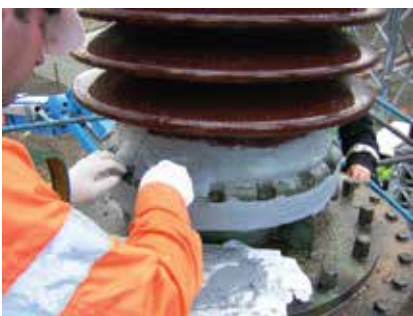
Brushing over the impregnated terylene strip
