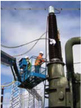
Cleaning the sealing surface
