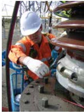
Applying the impregnated terylene strip
