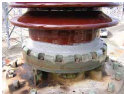
Finished overall profile
