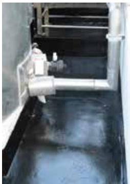
First coat of Belzona® 5811 (black colour).
