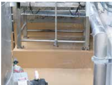
Belzona® 5811 reaches full chemical resistance after just 5 days cure time.
