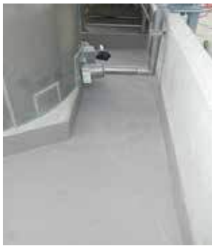
Bund area re-profiled with Belzona® Magma Quartz.
