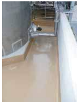
Bund area receives final coat.
