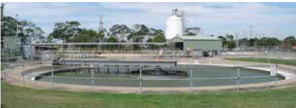
The clarifier to be repaired.
