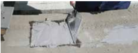
The Magma Quartz being applied.
