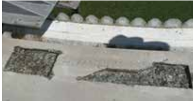
TX Conditioner applied by brush.
