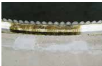
The repaired areas of the clarifier.
