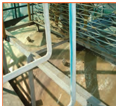
Vessel top view - before works
