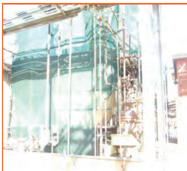
Curtained off - ready for blasting
