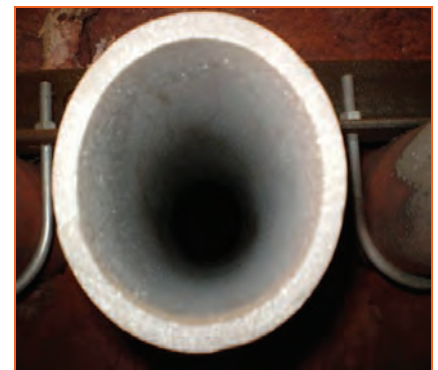
View with coke removed, after blasting with Sponge-Jet
